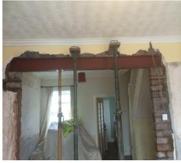
This usually undertaken. will be done (domestically) by using acrow props and strong timber needles. Alterations can be similar fashion made in however, commercial projects, stronger supports may be required by using super props. For this article though, we will assume that any structural alteration is to a domestic dwelling.
