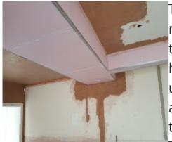
The support acrow props will stay in until the next day to let the mortar set. Only after this can the props be taken away and in doing so, any holes are filled with bricks and slate and pointed up as required. The plaster work is made good afterwards and any plasterboard encasement of the steel beam is done with fireline plasterboard. The building control officer will want to inspect all
